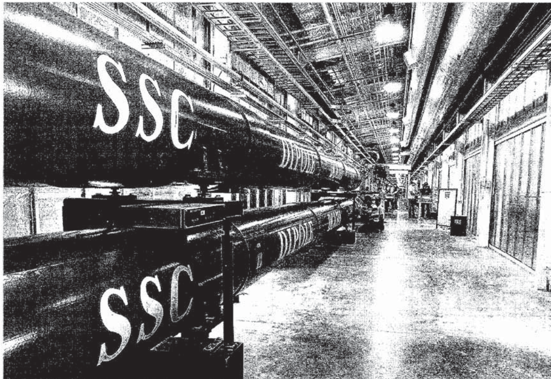
SSC dipole magnets on test, with the cryostat tubes mounted one above the other to simulate what the collider would have looked like.
